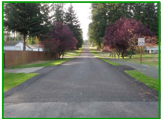
Realignment of East Price Street also eliminated deep ditches and short steep driveways. Widening the street and constructing a pedestrian path create a safer, friendlier roadway.
