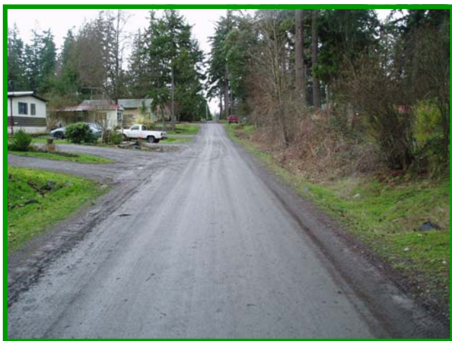
The narrow East Price Street road prior to improvements was frequently muddy in the fall and winter and dusty in the warmer months.
