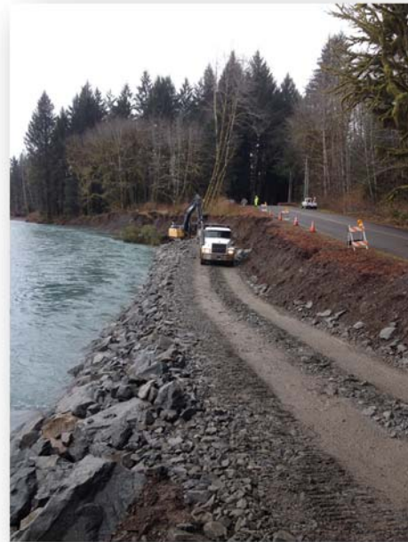
Upper Hoh Road MP 9.7 – Repair Underway
