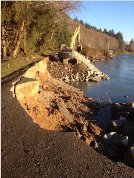
Oil City Road MP 8.8 – Repair Underway
