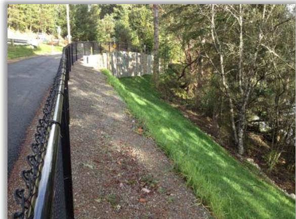
A soldier pile wall was constructed along a steep grade to allow room for the trail.
