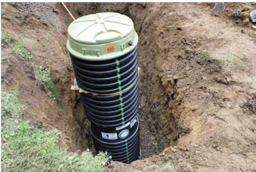
*Figure 4: Grinder pump being installed.*
