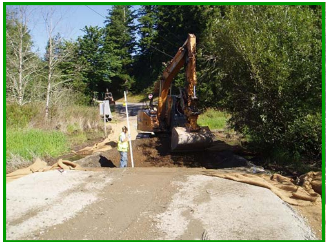
2. The old road bed was excavated to install five new culverts.
