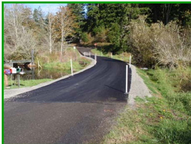
4. Asphalt surfacing completed the successful repair.
